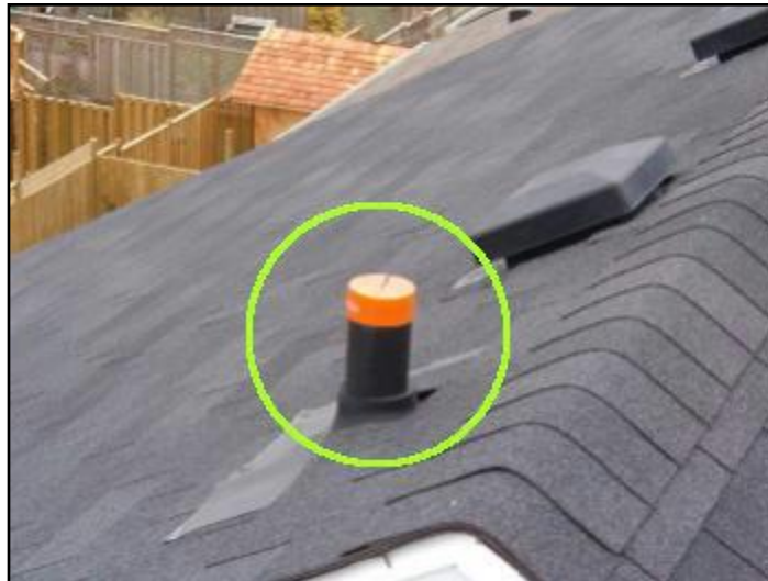
15. Plumbing stack is capped
