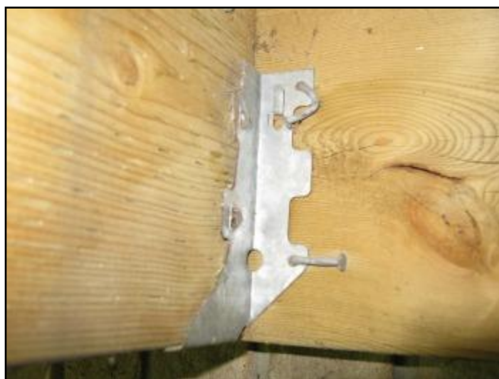
4. Poor end bearing, joist hanger connections
