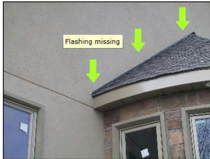
1. No kickout flashing at roof/sidewall junction
