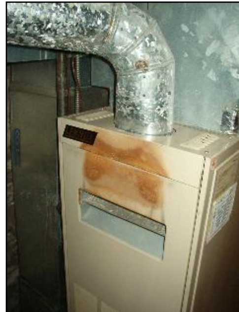
10. Evidence of furnace backdrafting
