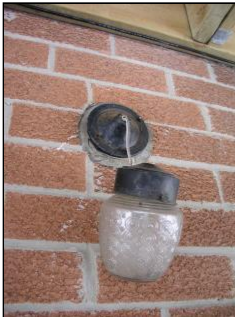
8. Light fixture is not well secured
