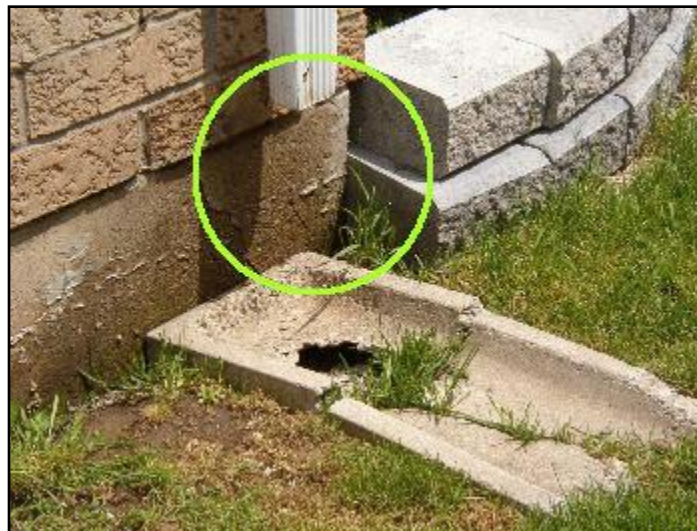
3. Downspout ends too close to building
